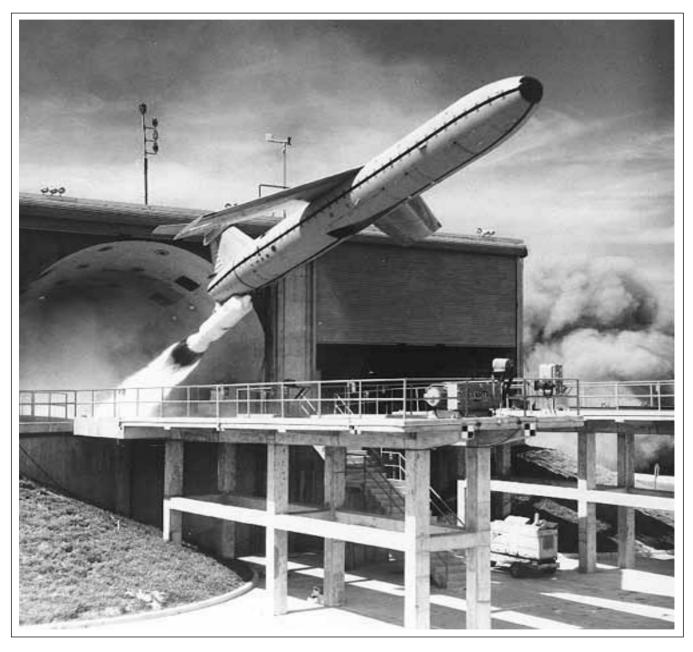
Developed in 1954, the Mace, like its predecessor, the Matador, was a tactical surface-launched missile designed to destroy ground targets. The Mace could be launched from a mobile trailer or bomb-proof shelter. It was propelled by a solid-fuel booster rocket that fell away following takeoff and was then powered up to speeds of 650 mph by a J33 engine. The first version created, known as Mace
